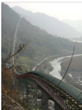
Picture 2: The pipe conveyors that can navigate curves allow bulk material to be transported in an environmentally friendly way, compared to transport on lorries.
