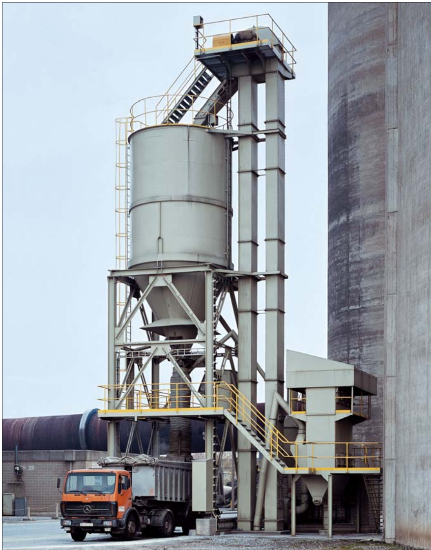
Dust-free loading of open vehicles with Portland cement clinker
