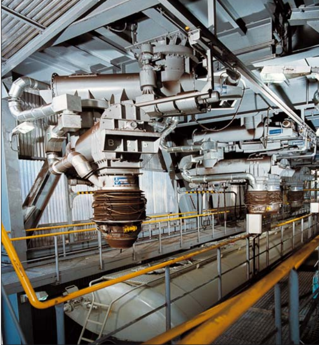
Cantilever double mobile articulated screw conveyor
