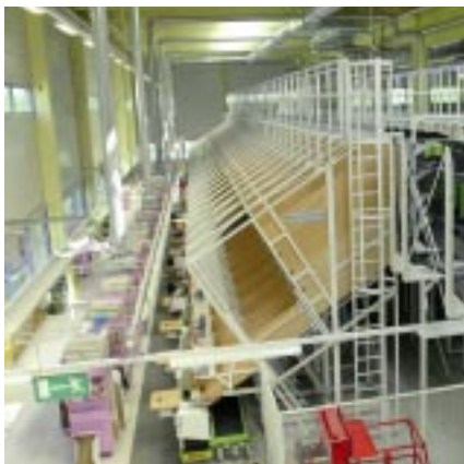
Several 4-level chutes are assigned to a packing station
