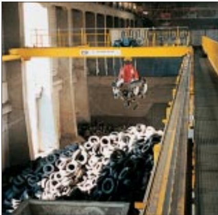
Storage bin with filling pit and discharge bin
