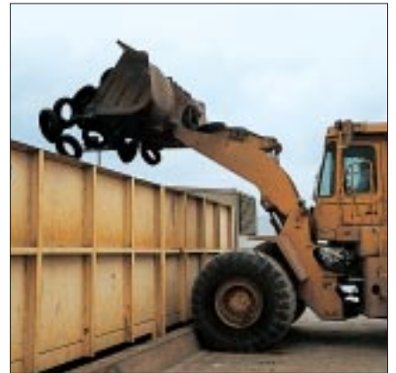
Supply box as an alternative to the storage area with filling pit
